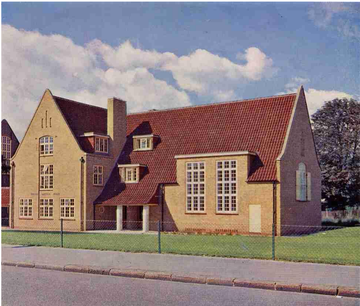
Figure 5: The 1956 meeting house as newly-built (photograph held at meeting house)
